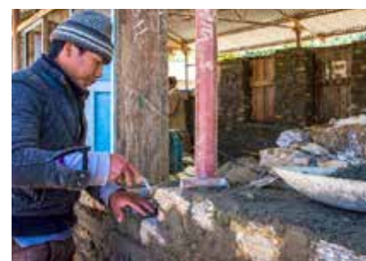
Construction underway at Garma School
