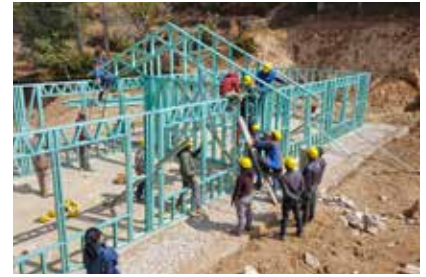
New construction after the earthquake at Garma
