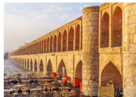
Siosepol, or Bridge of 33 Arches, constructed in 1602.
