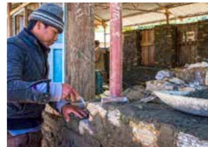
Construction underway at Garma School
