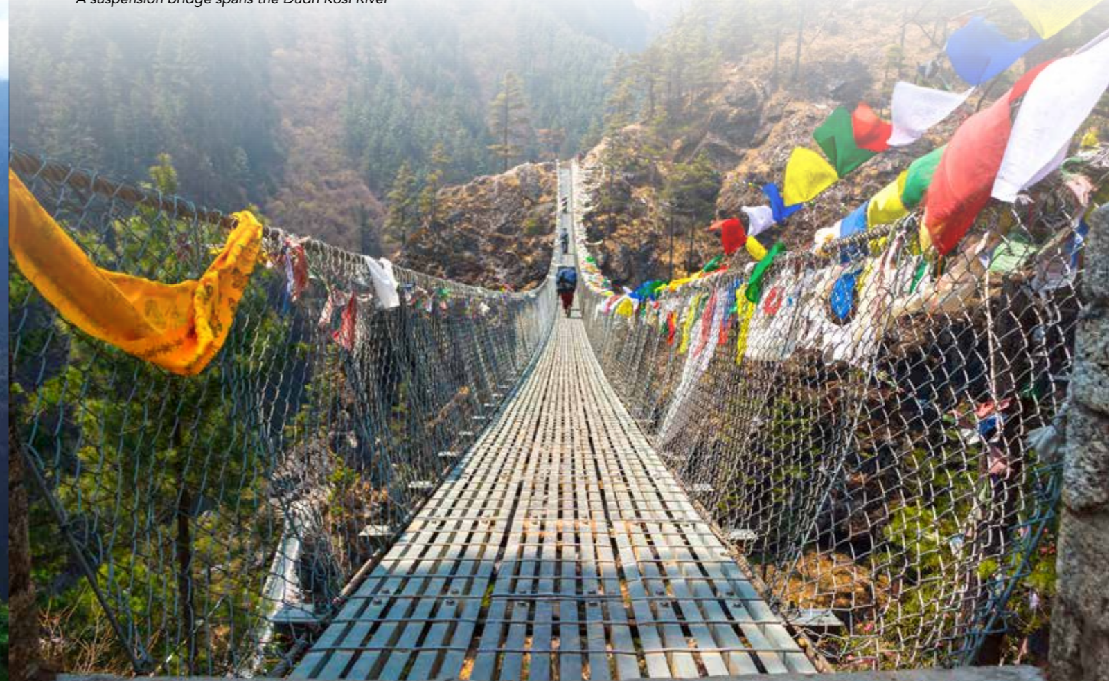
A suspension bridge spans the Dudh Kosi River
