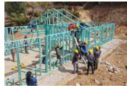
New construction after the earthquake at Garma
